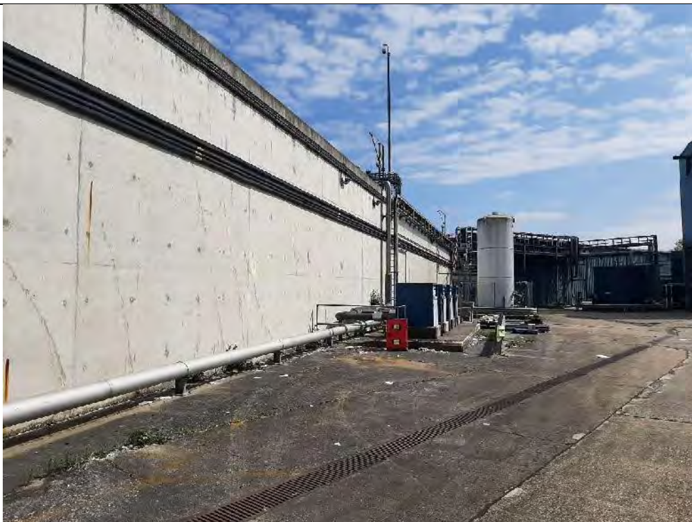
6. Effluent Treatment Plant Looking SE.
