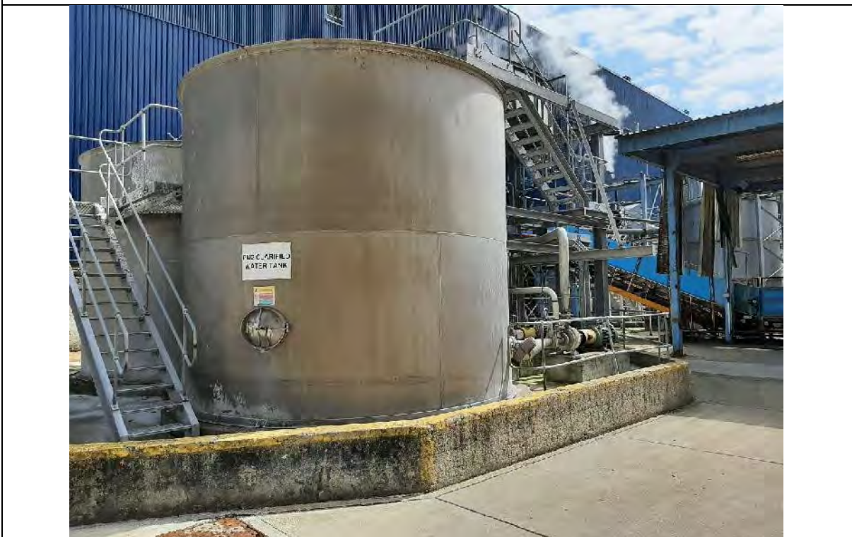
8. Water storage tank in southern area looking E.
