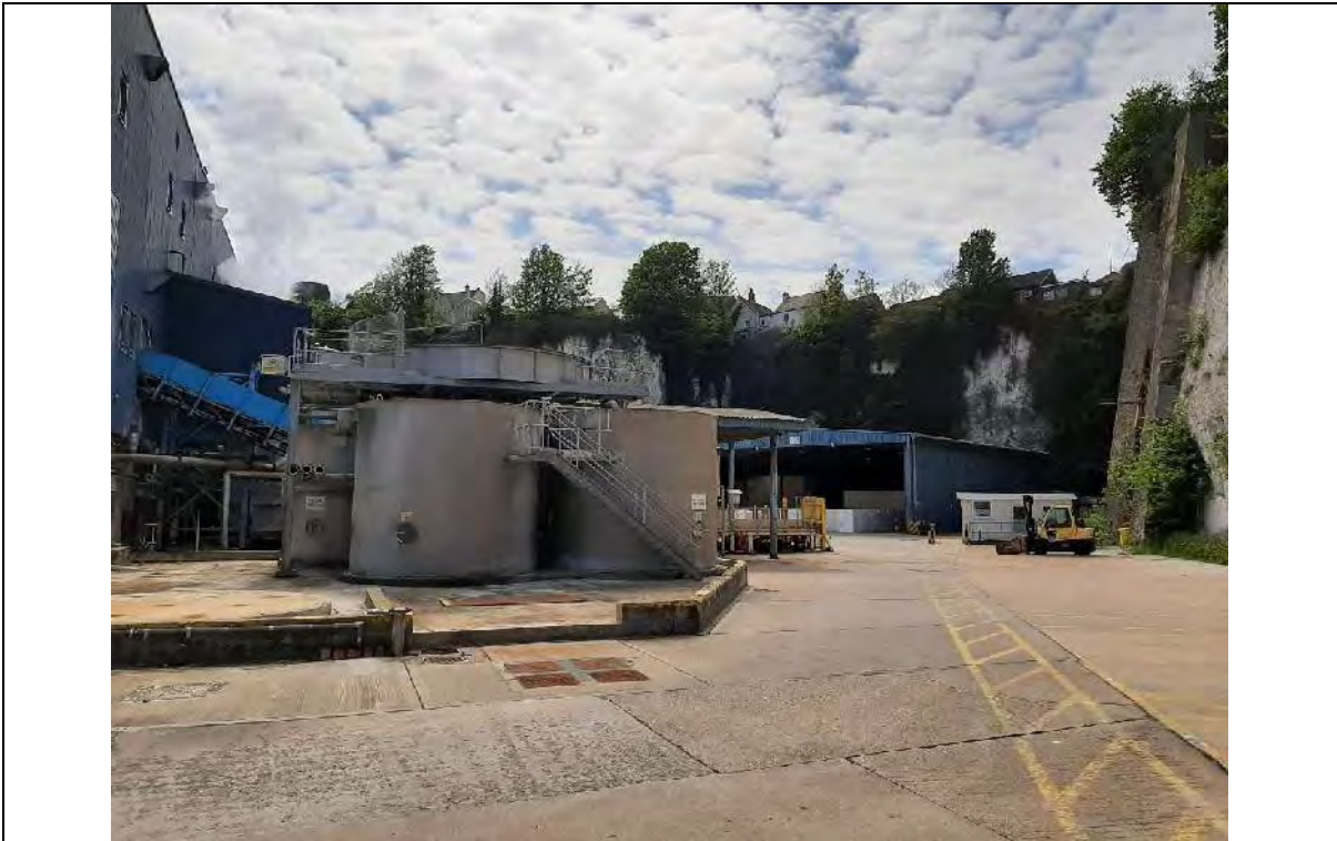
7. Storage tanks in southern area looking SE.
