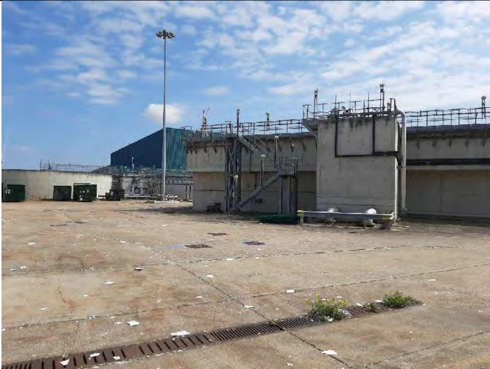
5. Effluent Treatment Plant Looking E.
