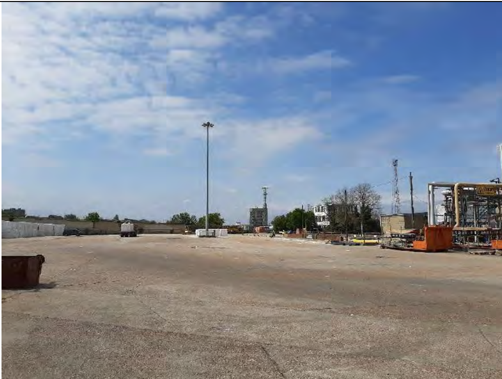
9. Proposed Development Area Looking W, south of the Boiler House.
