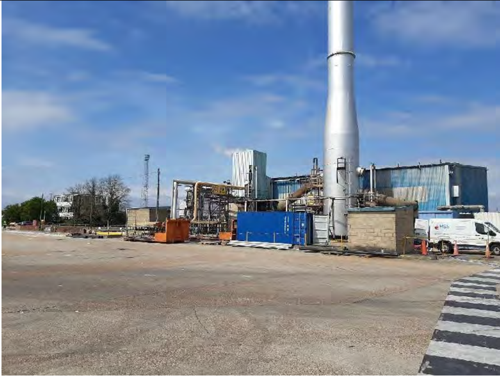
1. Boiler House Looking NW.
