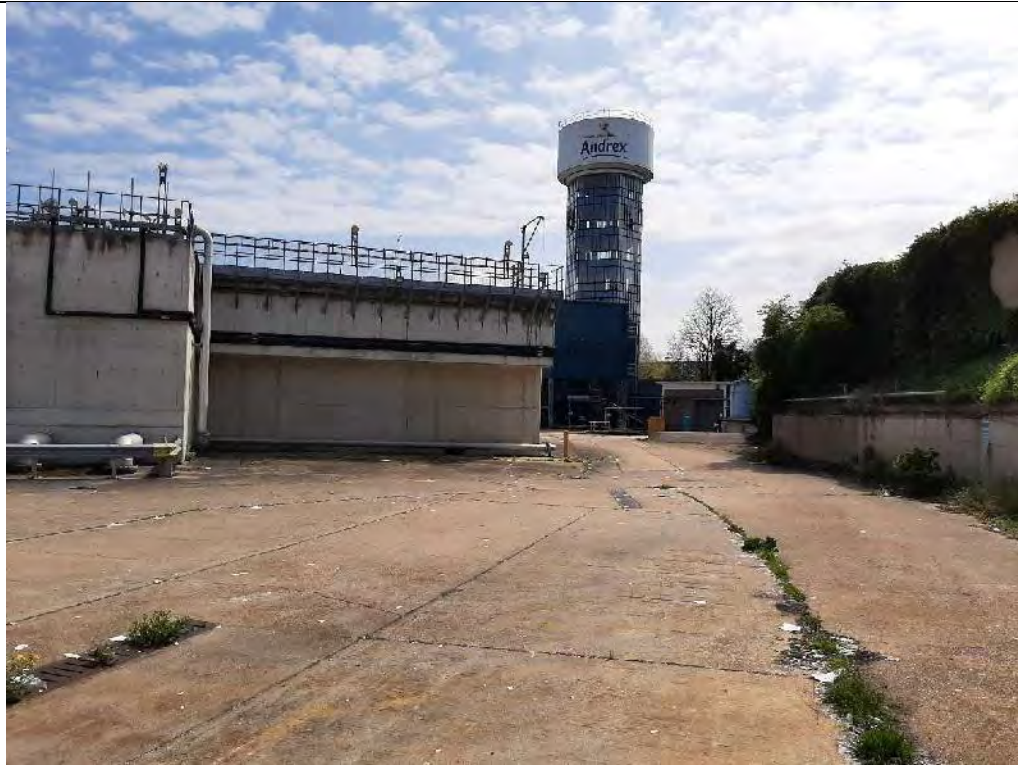
4. Effluent Treatment Plant and Water Tower.
