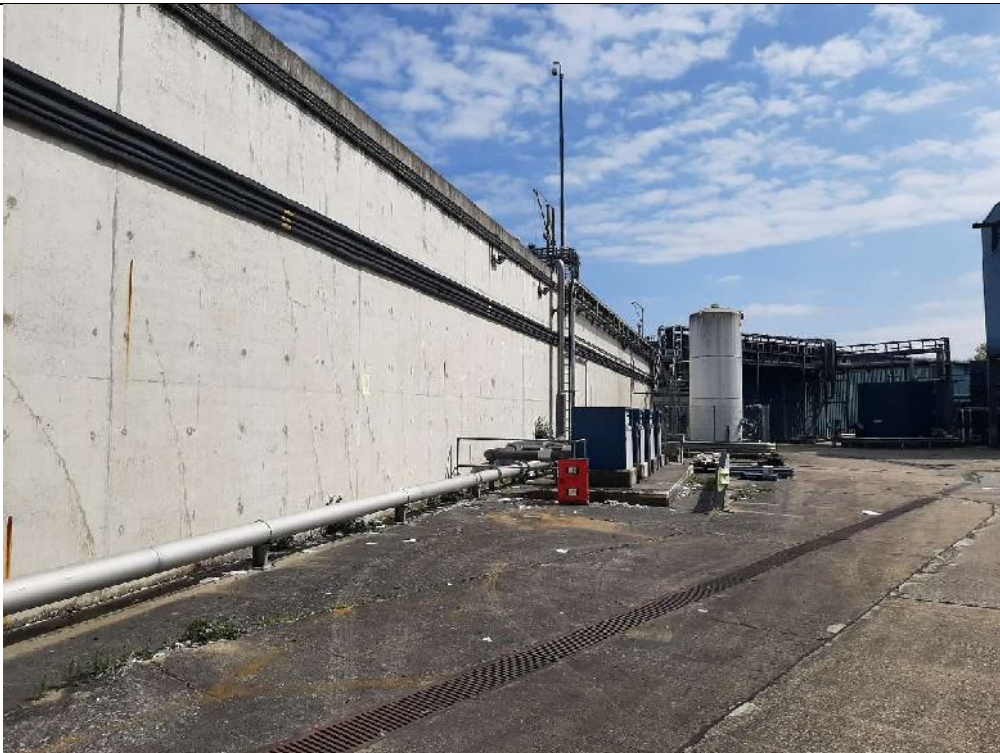
6. Effluent Treatment Plant Looking SE.
