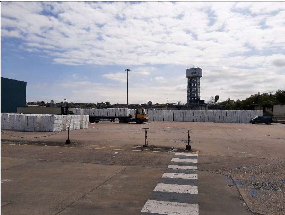
10. Proposed Development Area Looking S towards Effluent Treatment Plant.
