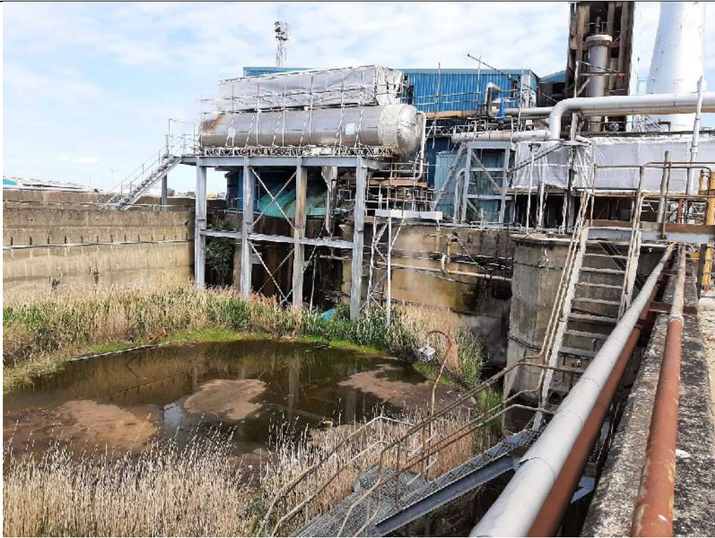
3. Boiler House Looking E showing one of the former sunken storage tank bases (former gas oil for the boiler house). The boiler house is now fired by natural gas.
