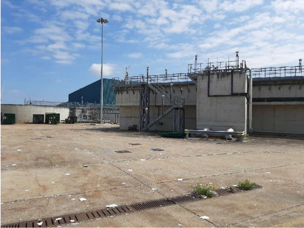
5. Effluent Treatment Plant Looking E.
