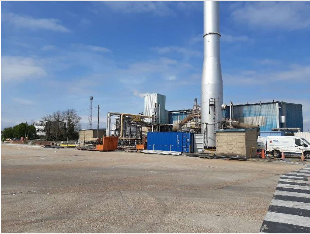
1. Boiler House Looking NW.
