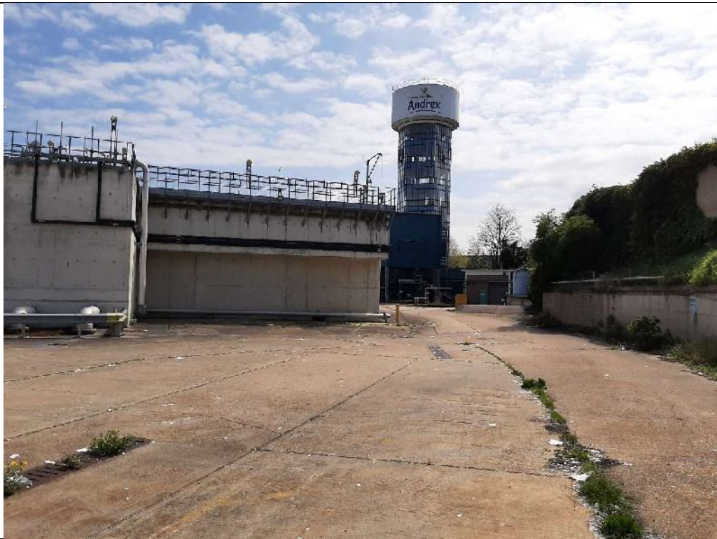
4. Effluent Treatment Plant and Water Tower.
