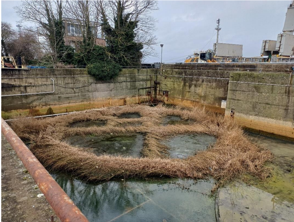
Standing water located to the north of the Site within the Study Area.
